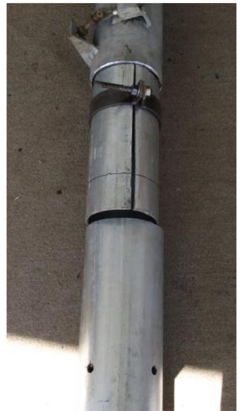
The sleeve clamped & inserted
