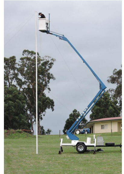
Preparing one of the four poles
