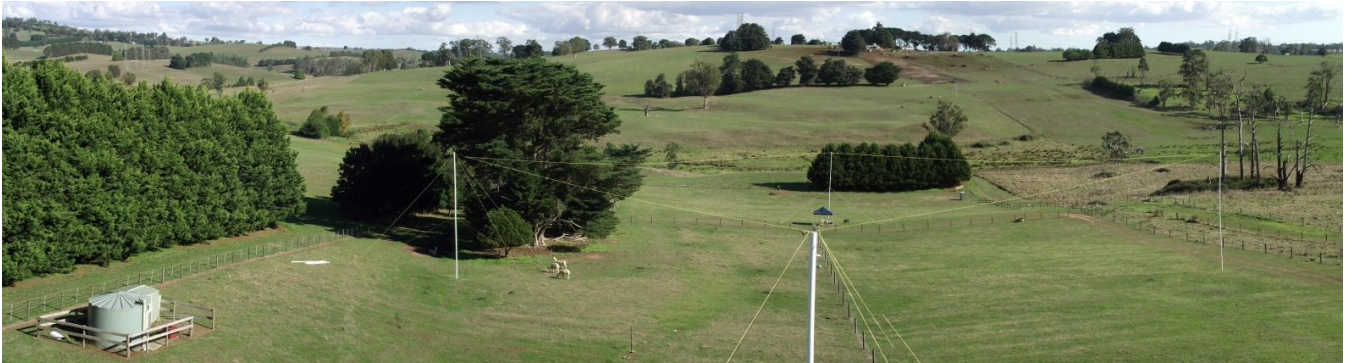
The Rhombic viewed from behind the terminating resistor. The position of the radiating wire has been digitally enhanced, as it would otherwise be invisible
